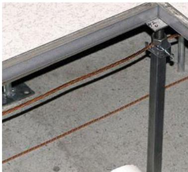
Figure 4. Ground wire in subfloor
